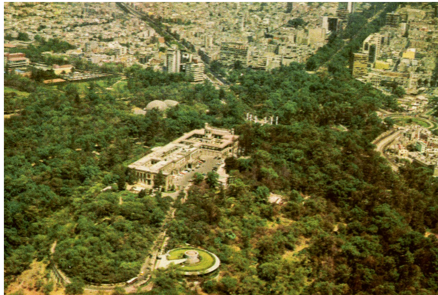
The vintage postcard features an aerial view of Chapultepec Castle. Sitting high amid the greenery – its elevation rivaled only by the nearby glass and metal skyscrapers – it remains a strange sight to behold. An image suspended in time.
